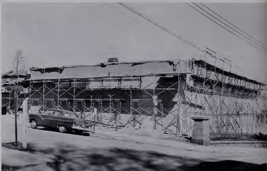
Meriden Boys' Club (Under construction in 1956)
